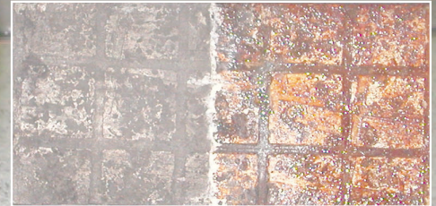
After Applying Vapro 812
